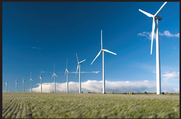
Big Horn Wind Power Project, Washington
