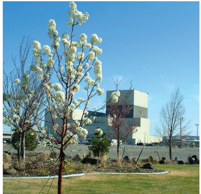
Columbia Generating Station
