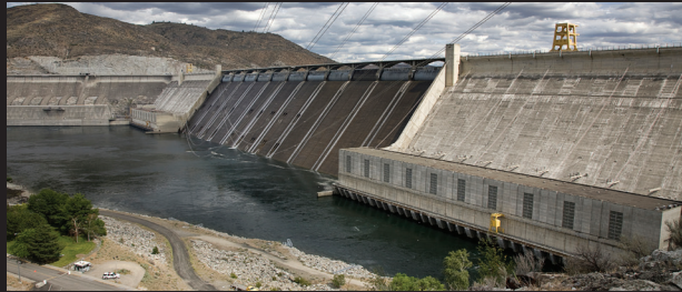
Grand Coulee Dam, Washington
