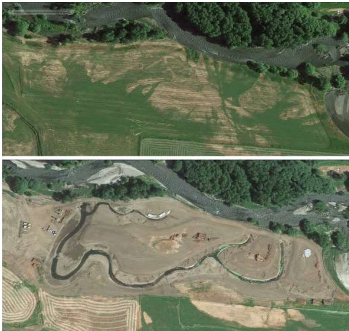
Figure 11 Short-term impacts to a floodplain during restoration project showing conditions before (upper photo) and during (lower photo).
