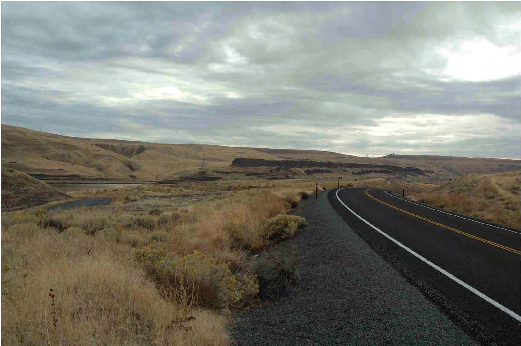
Figure C-9c shows the simulated view of a routing alternative segment common to all action alternatives from Viewpoint 9.
