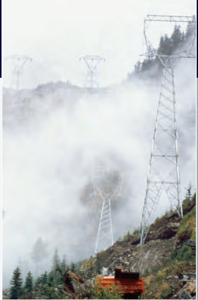
A fire burning under a power line can create a dangerous situation. Stay away from lines if a fire is nearby.
