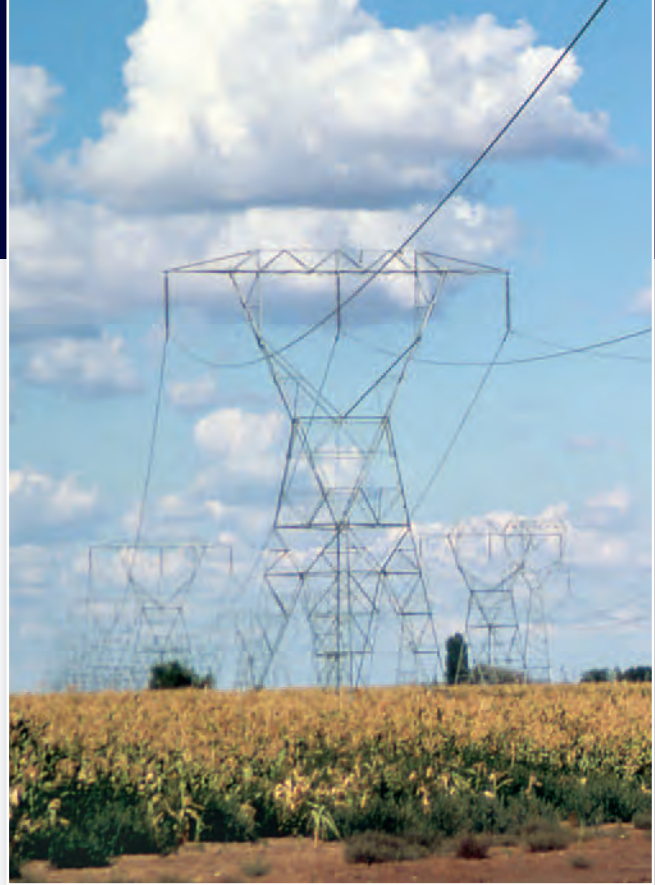
Most crops, less than 10 feet in height, can be grown safely under power lines.
