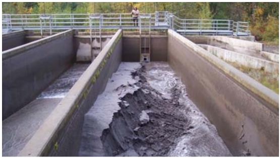
Source: East Fork Irrigation District, photographed in 2010 Figure 1-5. The District's sand trap facility located 0.4 mile from the diversion at the start of the Main Canal.
