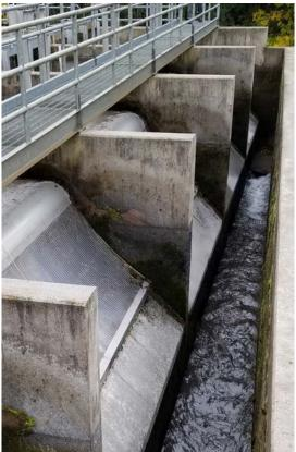
Source: Hood River Watershed Group Figure 1-6. Coanda type fish screens installed at the end of the District's sand trap settling bays.
