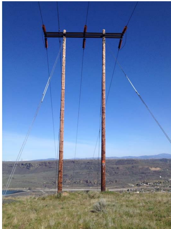
Figure 3-23. View of Structure 3/4 and Buttes in the Distance
