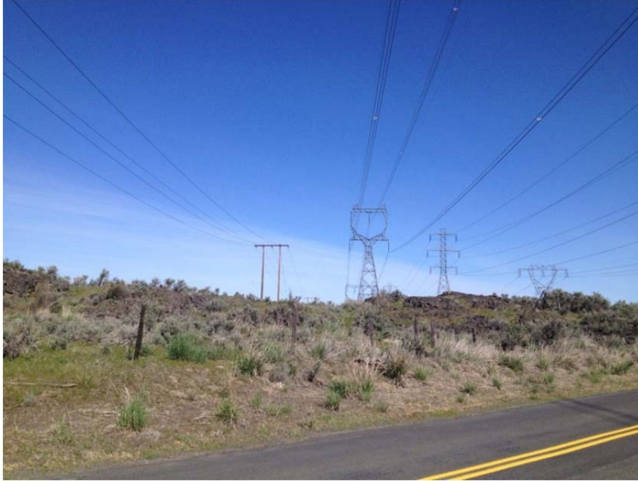
Figure 3-24. View of Structure 4/2 from Grand Coulee Hill Road
