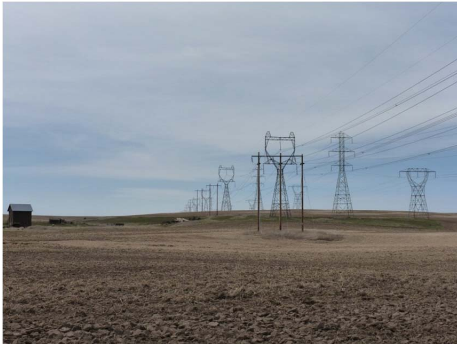
Figure 3-26. Looking North at Structure 24/3
