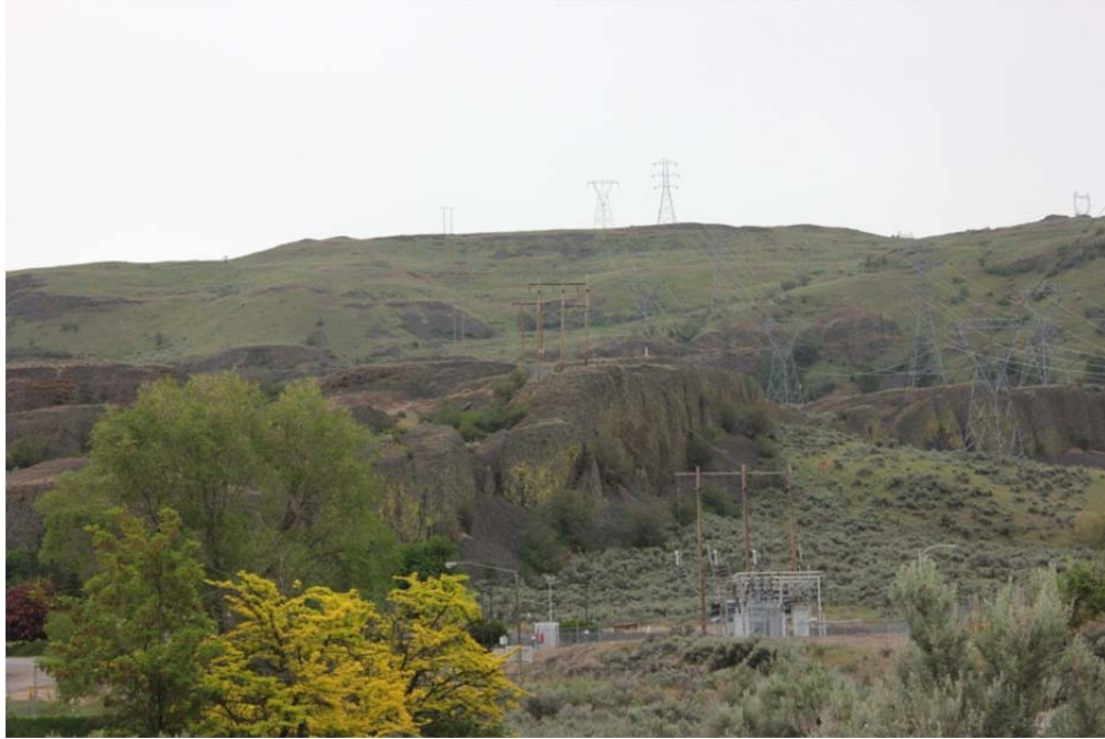
Figure 3-16. Cliffs and Caves near Structure 2/6
