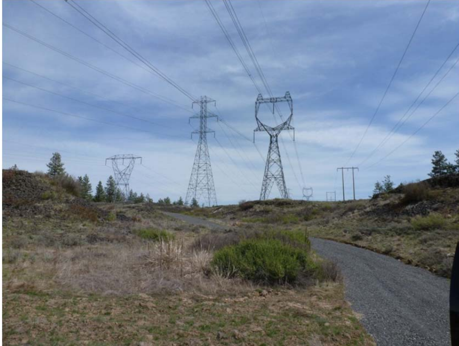
Figure 3-27. Looking South at Structure 28/4
