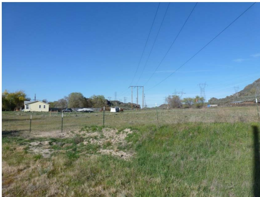
Figure 3-19. Looking South with a View of Residences and Pastures near Structure 1/5
