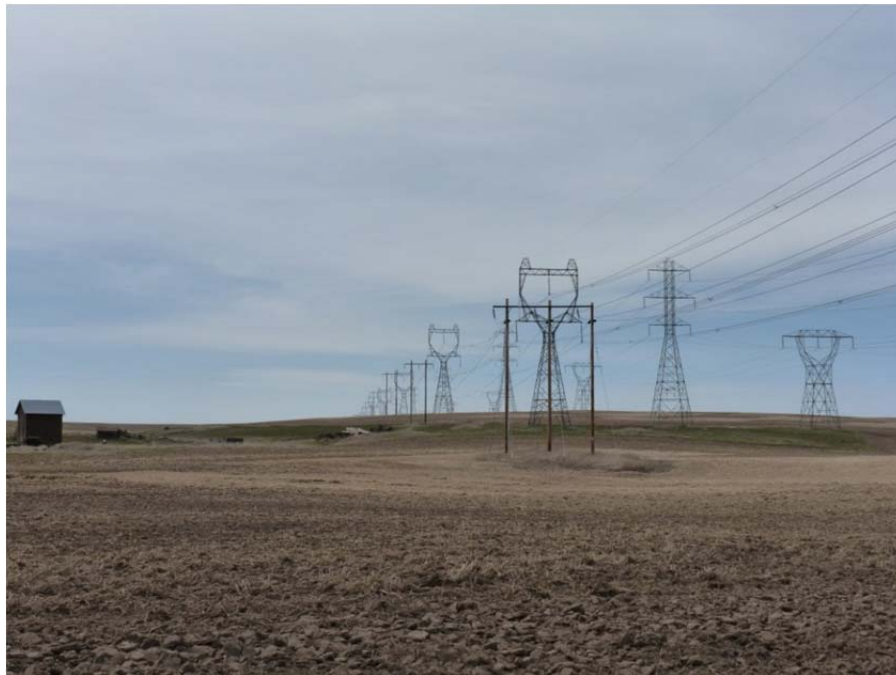
Figure 3-18. Looking North at Structure 24/3
