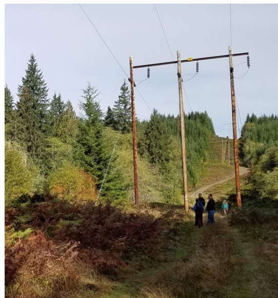
Figure 2-2. Existing Three-Pole Wood Structure
