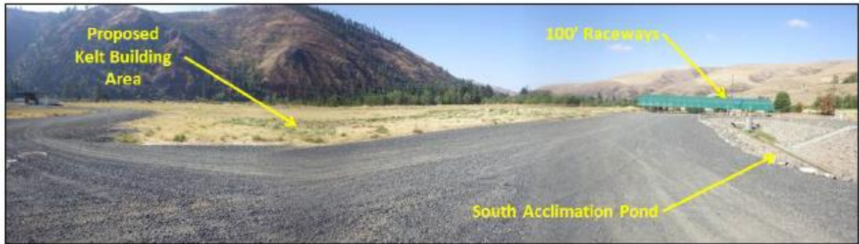
Figure 6 Location of proposed kelt reconditioning facility within the current hatchery complex
