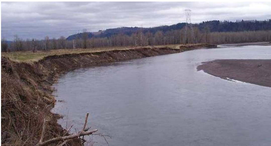
Figure 17 - Emerging Meander in the West Channel Showing the Severely Cut Bank, looking upstream
