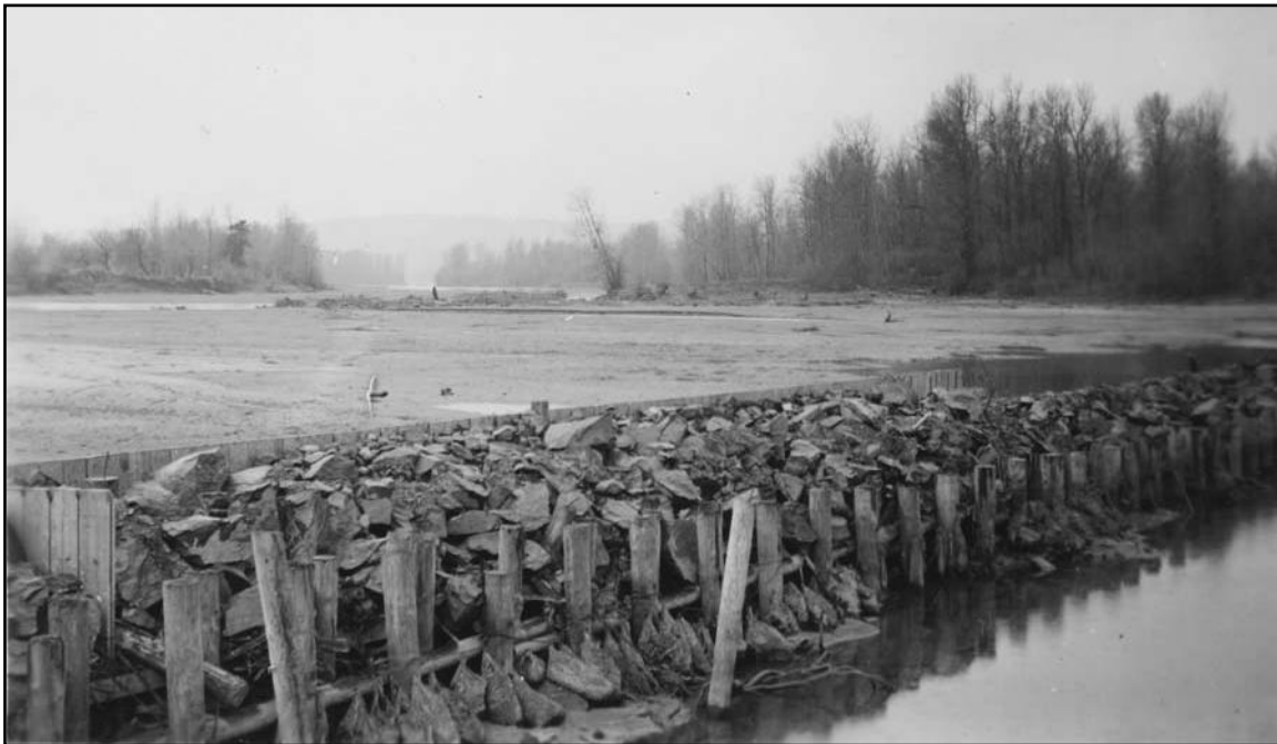
East Channel Dam under Construction, Sandy River Delta, 1930s
