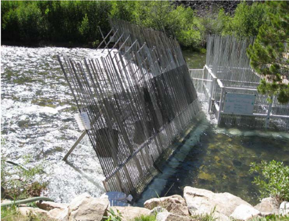
Figure 7. Existing weir on Yankee Fork
