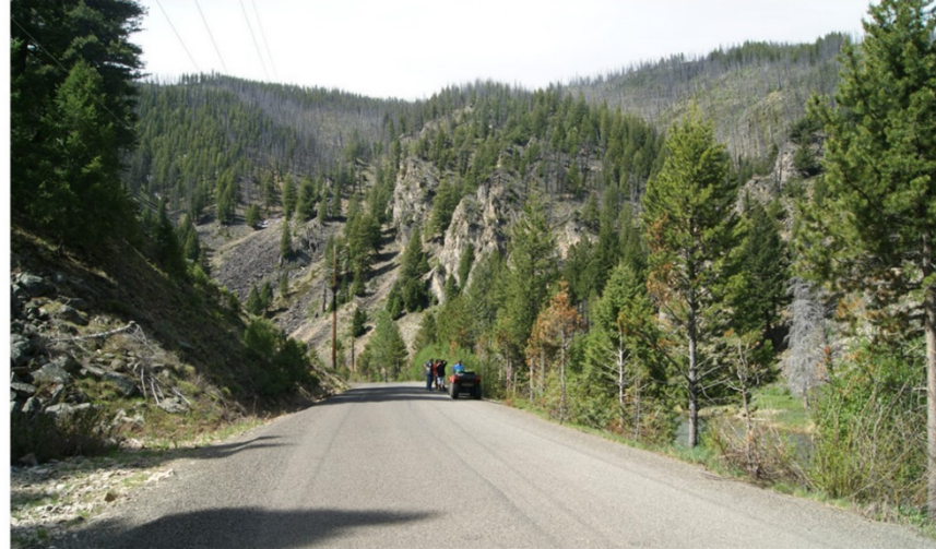
Photo 2. Looking south from Yankee Fork Road, south of the proposed satellite facility, toward the bend in the road.
