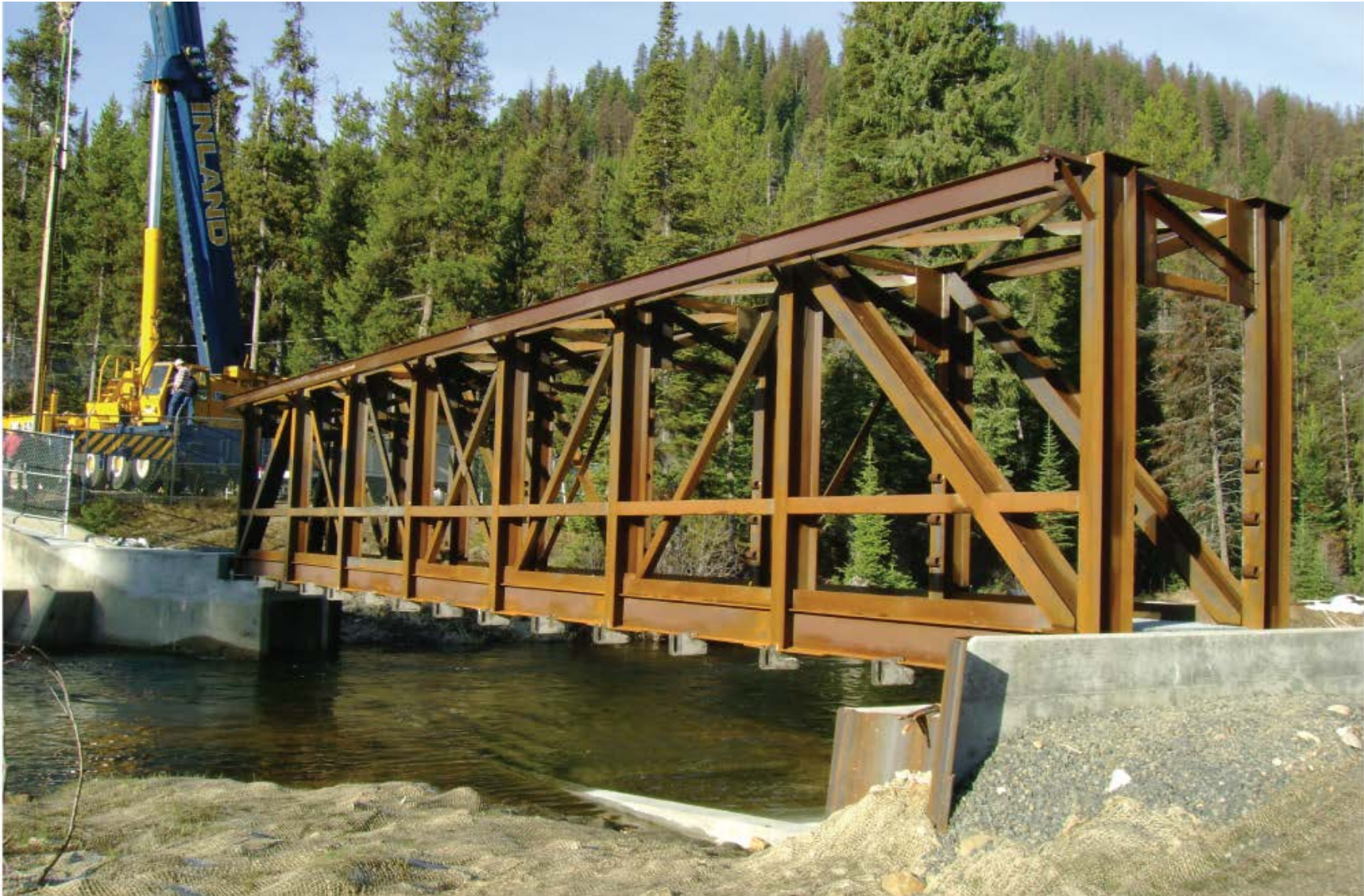
Figure 2-6a. Example of Bridge Weir Fully Constructed (South Fork Salmon River Bridge Weir)
