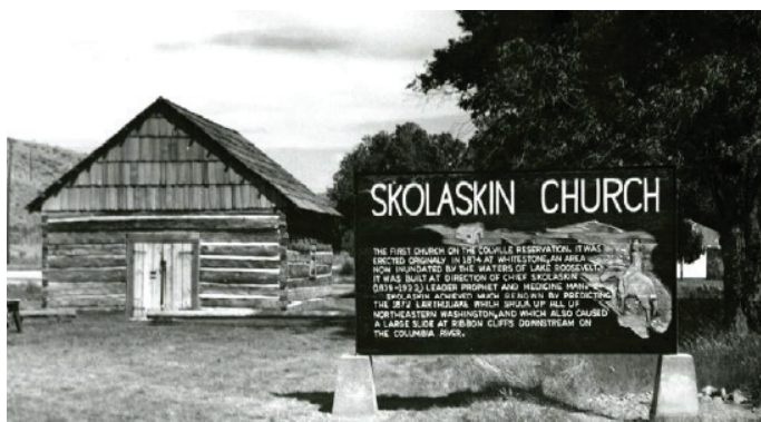
Skolaskin's Church rehabilitation, Grand Coulee Project, completed FY 2018.
