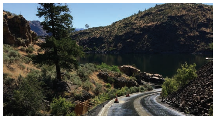
Rock image stabilization project at Lake Roosevelt, Grand Coulee Project, FY 2017.
