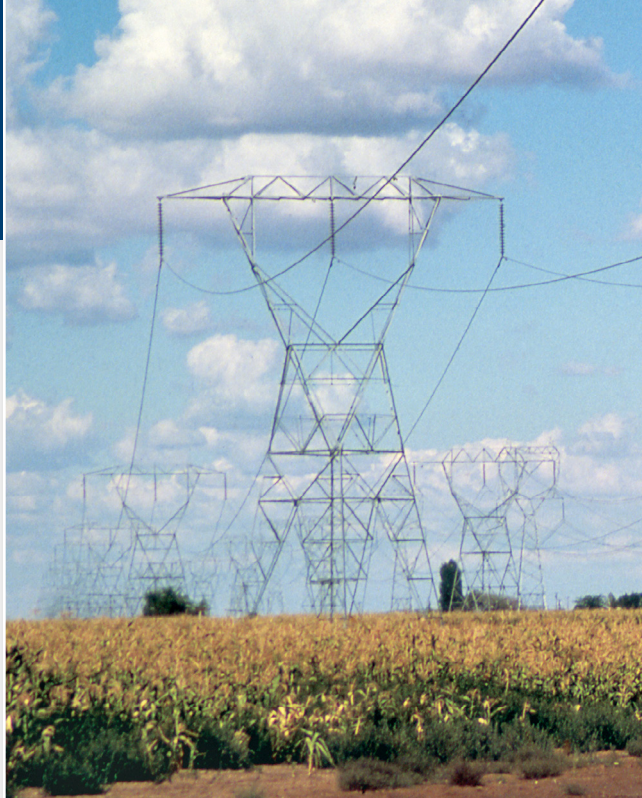
Most crops, less than 10 feet in height, can be grown safely under power lines.
