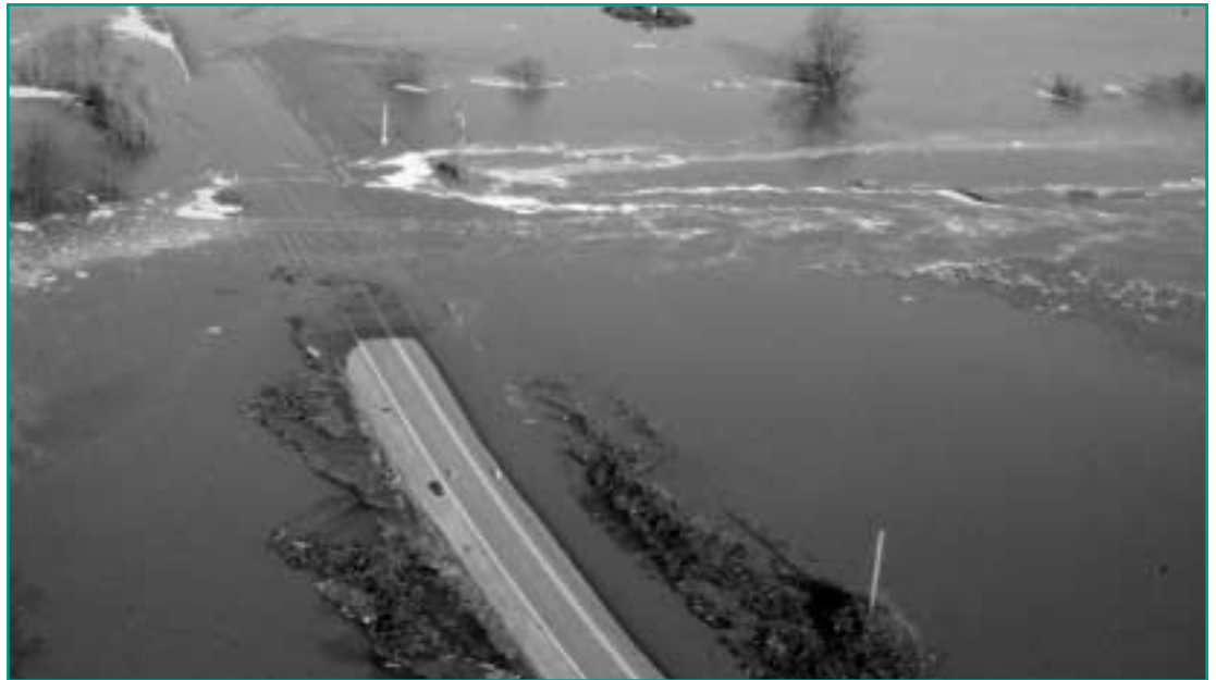
Levee systems provide another method of flood protection. There are over 20 levee systems in the lower Columbia River, and, in high water years, they add another layer of security for residents in flood prone areas.
