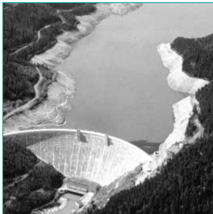
Hungry Horse Dam is an important component of the region's power generation system, turning water into kilowatts of electricity.
