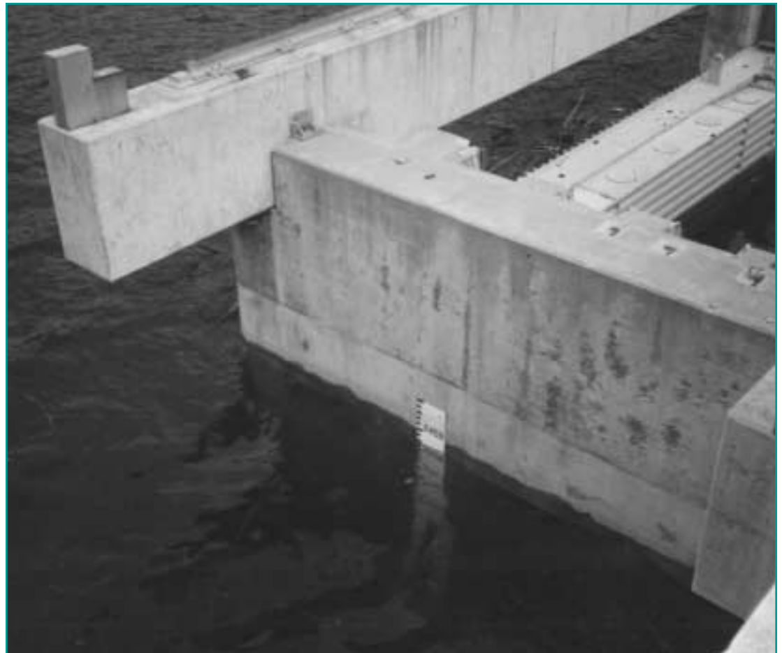
Indicators, like this one at Libby Dam, are used to gauge the water level at each reservoir. Efforts are made to refill the reservoirs every year. Runoff is usually adequate to refill reservoirs about three out of every four years.
