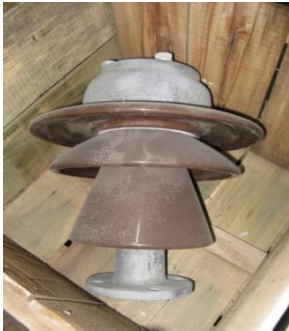
33 kV Pin Insulator
